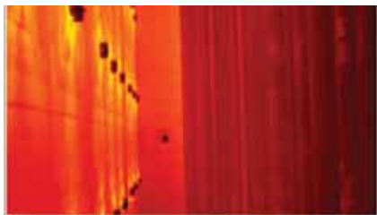
Pipe with high thermal stress in reformer plant used for production of ammonia. Photo courtesy of Haldor Topsøe A/S.
