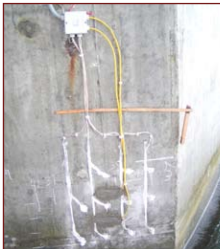
CorroRisk mounted on a bridge pillar
