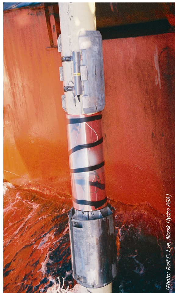
The diode package installed to the sacrificial aluminum anode and the connection to the cathode plate
