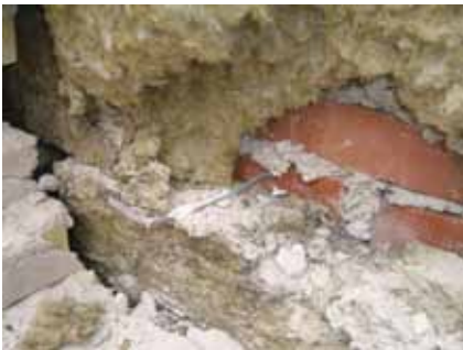
Housing association Fjordblink. Almost intact tie can be seen. Photo courtesy of Grontmij A/S in Aalborg.
