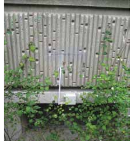
Measuring of corrosion rate with and without applied inhibitors
