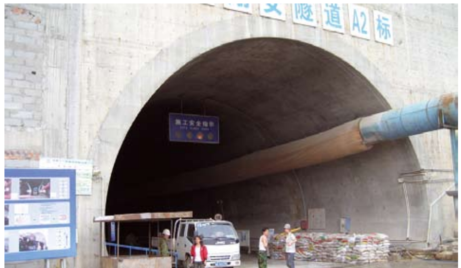
The entrance to the new Xiang'an tunnel.
