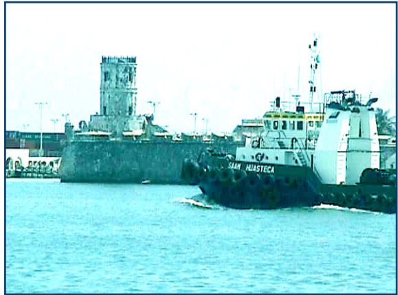
From the port system transformation, the Veracruz port has shown great advances in productivity and installed capacity
