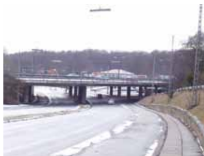
Figure 1: The Skovdiget Bridge
