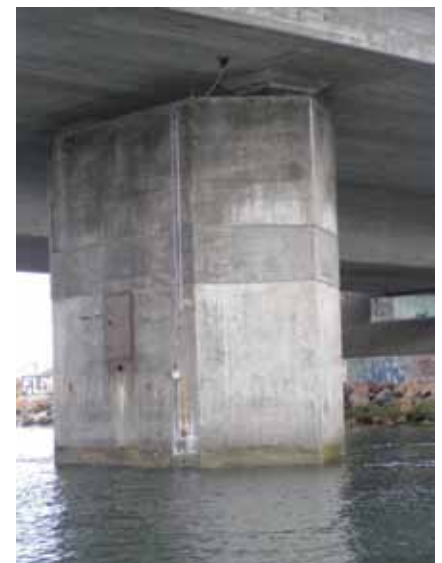
Figure 5: Close-up of the installation of CorroRisk sensors.
