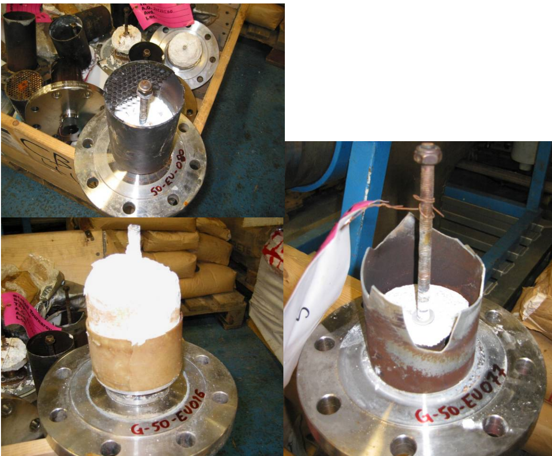
Picture 4: Flange mounted anodes with damaged and missing covers
