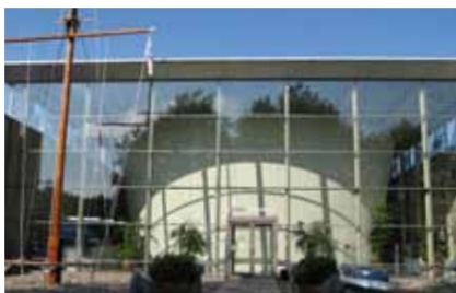
At our facilities in Lyngby, Denmark, we offer training and port studies in our seven full-mission and part-task simulators and testing and design evaluation in our towing tanks and wind tunnels.
