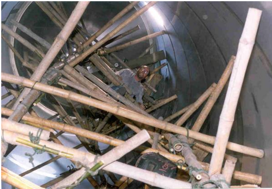
FIGURE 6 – Overview photo showing the magnitude of the repair work.
