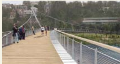
View of the foot bridge's deck.
