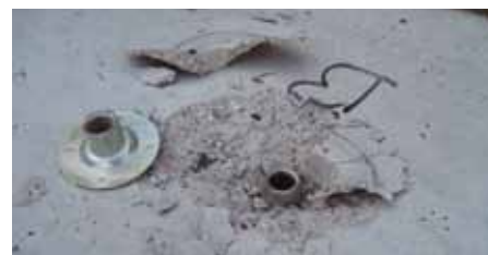
Fracture in anchor as a result of tensile testing.
