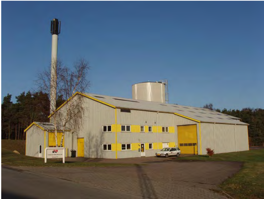
The heating plant with straw storage to the right, boiler building in the center, stack to the left, and the heat storage tank behind
