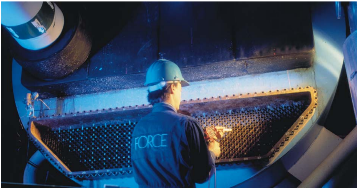
Heat Exchanger Inspection by FORCE Technology
